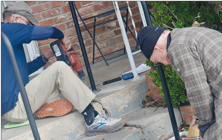
Safe at Home volunteers Dan Ward, of Carmichael, and Stan Jones, of the Greenhaven/Pocket area, install a handrail for a Sacramento resident in need of safer step way. Photo courtesy of SAFE Credit Union
